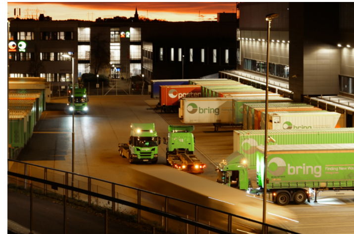
Posten Norge and Bring's logistics centre in Oslo is being expanded to grow in step with the market
